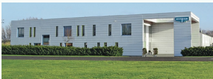
EVAPCO Europe A/S, Aabybro, Denmark
