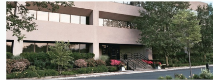
EVAPCO Dry Cooling, Bridgewater, New Jersey
