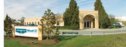
EVAPCO Alcoil, York, Pennsylvania
