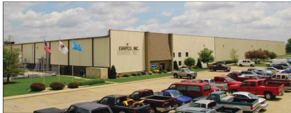
EVAPCO Trung Tây, Greenup, Illinois
