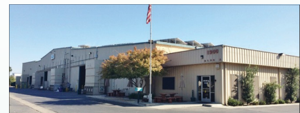
EVAPCO West, Madera, California
