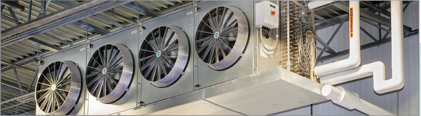
SSTME Evaporator with long-throw adapter
