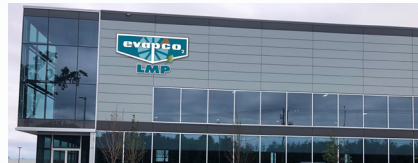
EVAPCO LMP, Laval, Quebec
